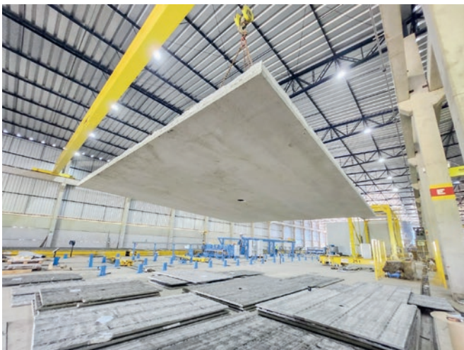
The precast elements are manufactured and transported using software-controlled systems, some of which are fully automated – this saves time and money and makes production safer.
