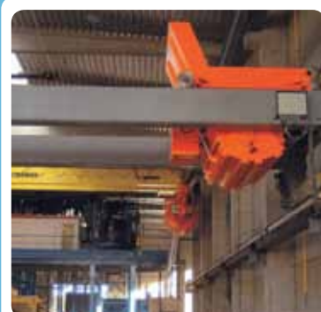
Rollover bucket and concrete distributor
