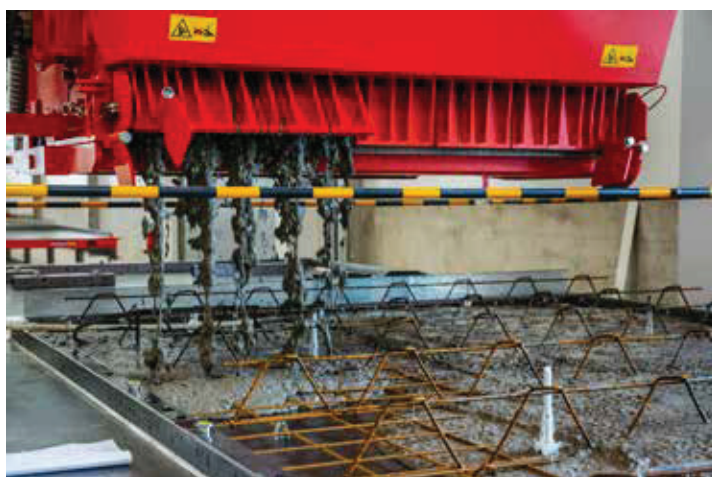
Thomas Betong is producing double walls in their carousel plant in Heby for housing projects in Stockholm
